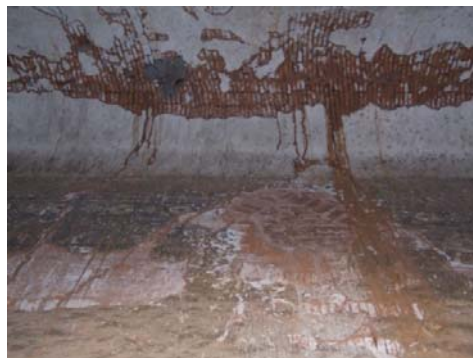
1499 MIN-NYEIN-KON. SWALLOWS' NESTS (UPPER LEFT SIDE OF PHOTOGRAPH) AND MUD RUN-OFF (RIGHT SIDE) DUE TO WATER INFILTRATION DISSOLVING CONSTITUTIVE MUD-BASED MORTAR AND DEPOSITING ELSEWHERE.
