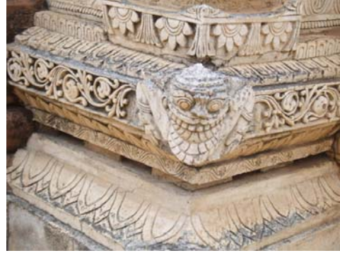
1825 TEMPLE, DETAIL OF STUCCO MOULDINGS THAT SHOW TRACES OF DECAY WHERE RAIN STRIKES ON HORIZONTAL SURFACES.
