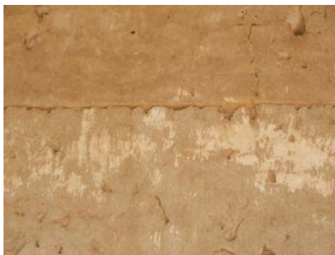
2162 ANANDA-OK-KYAUNG MONASTERY, AFTER THE APPLICATION OF A RENDERING LAYER, THE HORIZONTAL LOWER BORDER WAS COMPRESSED WITH A SLANTING ENDING SO AS TO APPLY BY OVERLAPPING THE SUBSEQUENT LAYER.
