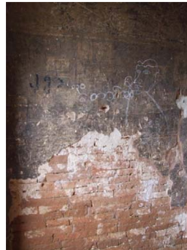
433 PYWAN-TAN-HSA-HPAYA. LACUNAE OF PLASTER IN-DEPTH SHOWING THE BRICKWORK, COMBINED WITH SUPERFICIAL ONES THAT ARE THE REMAINING WHITE PLASTER.
