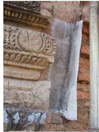
539 TAYOK-PYI-HPAYA-GYI, TEMPLE UPPER STOREY, NORTH FACE, EAST SIDE OF PORCH. SECTION OF RENDERING FACED WITH COTTON GAUZE AND HIGHLY REVERSIBLE GLUE.
