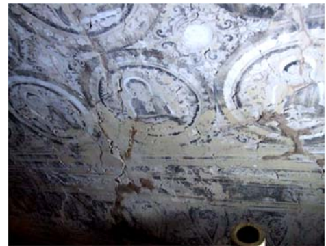
1847 (HPAYA-NGA-ZU GROUP), CROSSING CRACKS ON PLASTER, PROBABLY FROM DISLODGED BRICKWORK BENEATH.
