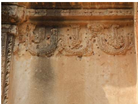
1812 HTI-LO-MIN-LO TEMPLE, EAST FACE, SOUTH SIDE. STUCCO MOULDINGS ANCHORED BY WOODEN PEGS INSERTED INTO THE RENDERING LAYER AND MASONRY.
