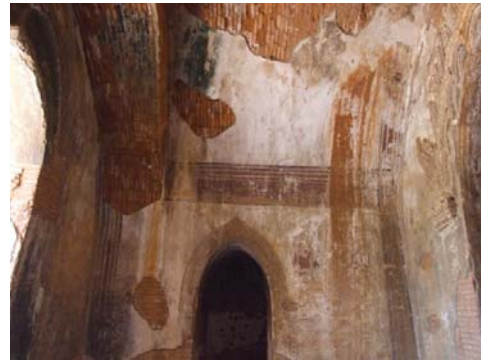
1457 MAHA-GU-GYI, VESTIBULE, SOUTH WALL MUD RUN-OFF THE SURFACE DUE TO INFILTRATION INTO THE MASONRY WASHING AWAY CONSTITUTIVE MUD-BASED MORTAR, AT THE LEFT GROWTH OF MICRO-ORGANISMS (ALGAE).
