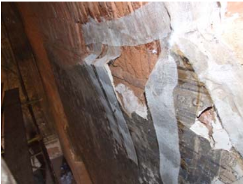
1471 THEIN-MAZI, VESTIBULE, NORTH WALL PROVISORY BANDAGE ADHERED SECURING THE SEVERELY DETACHED MURAL PAINTINGS.
