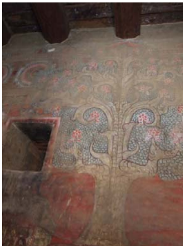
2162 ANANDA-OK-KYAUNG MONASTERY, SHRINE, EAST WALL. MURAL PAINTINGS COVERED AT THE TOPMOST WITH A THICK LAYER OF DUST WHEREAS THE LOWER SECTION SHOWS HEAVY DEPOSITS OF SOOT.
