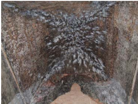
1202 ABEYA-DA-NA, CELLA, VAULT. BAT DROPPINGS ON THE VAULTING SURFACE.
