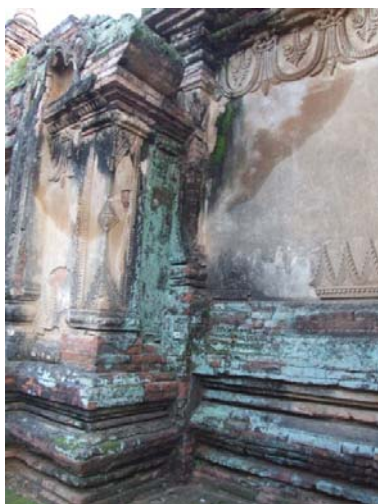
1323 KUBYAUK-GYI (MYINKABA), NORTH LATERAL FOREPART WITH WINDOW, WEST SIDE. ONGOING WATER INFILTRATION FROM UPPER PARTS GIVEN BY THE DARKER AREAS ON THE PLASTER, NOTICE THE DEVELOPMENT OF MICRO-ORGANISMS ON THE SURFACES.
