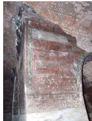
1969 PITAKAT-HPAYA, DUST DEPOSITS ON PROTRUDING SURFACES AS WELL AS DEVELOPMENT OF MICRO-ORGANISMS PERHAPS DUE TO WATER INFILTRATION FROM THE ROOF (THE BLACKISH UPPER SECTIONS).
