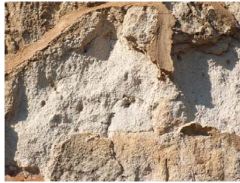
2162 ANANDA-OK-KYAUNG MONASTERY, UPPER STOREY, SOUTH FACE, PEDIMENT OF WESTERN DOOR. POWDERING STUCCO MOULDINGS DUE TO SALT RE-CRYSTALLISATION DUE TO WET-DRY CYCLES.
