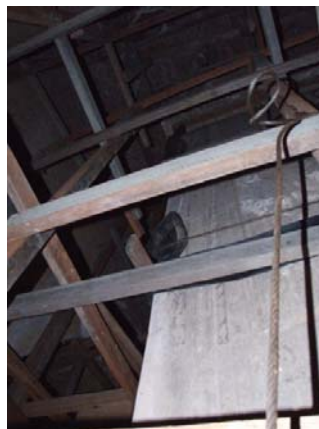
539 TAYOK-PYI-HPAYA-GYL, UPPER STOREY, SHRINE, SOUTH EAST CORNER OF CENTRAL CORE. THE STAINLESS STEEL BELT WAS INSTALLED ON A THIN BLACK RUBBER SHEET DIRECTLY SET ON THE PAINTINGS. THIS WILL CAUSE DAMAGE TO THE PAINTED PLASTER AT THE CORNER.
