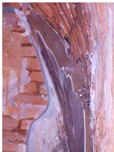
657 THAN-BU-DE-HPAYA. LIME RENDERING, MUD-BASED PLASTER, THIN LIME-BASED PLASTER.
