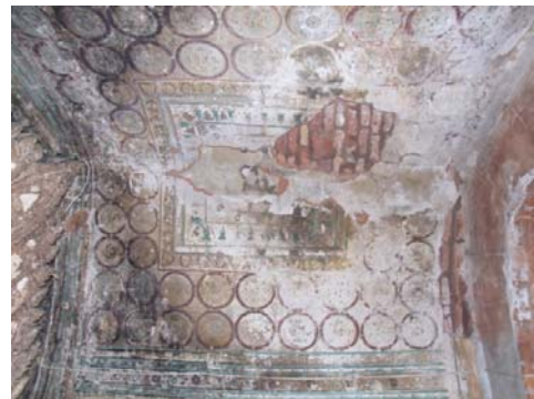
1336 TEMPLE, VESTIBULE VAULT. ALTERATION OF RED VERMILION INTO BLACK ON THOSE AREAS HIT BY REFLECTED SUNLIGHT WHEREAS, THE AREAS THAT ARE NOT UNDER THE SUNLIGHT REFLECTION ARE LESS ALTERED. WATER INFILTRATING HAS WASHED AWAY A GREAT DEAL OF PAINTING.
