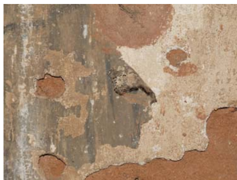
568 TEMPLE. LIME-BASED PLASTER & CLOTH ADHERED TO THE SURFACE WITH PRIMING LAYER.
