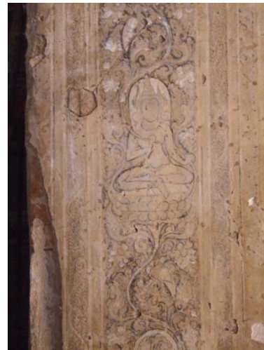
534 SA-PWE-TIN, CIRCUMAMBULATORY CORRIDOR. HEAVY OVER-CLEANING IN WHICH, THE PREPARATORY DRAWING OF THE CENTRAL FIGURE WAS REVEALED HAVING DELETED FOREVER THE PAINTING.
