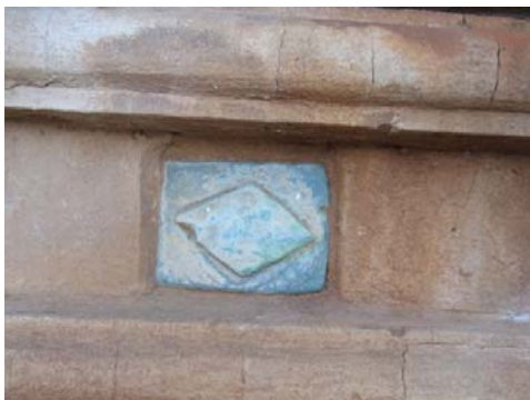
539 TAYOK-PYI-HPAYA-GYI. GLAZED PLAQUE WITH DEPOSITION OF CALCIUM CARBONATE MIXED WITH DUST ON THE SURFACE, THIS IS THE YELLOWISH FILM ON THE GREEN GLAZE.
