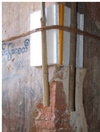
539 TAYOK-PYI-HPAYA-GYL. MODEL OF PROTECTION OF THE MURAL PAINTINGS OR STUCCO MOULDINGS WITH POLYSTYRENE SHEETING AND WOODEN PLANKS OR BEAMS BEFORE INSTALLING A STAINLESS STEEL BELT.
