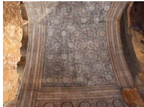
571 TEMPLE, SOUTH VESTIBULE, VAULT. THE CLEANING OF THE PAINTED SURFACE SHOWS NON HOMOGENEOUS APPLICATION OF SOLVENTS AND PERHAPS WITH DIFFERENT TIMING. DARK AND LIGHT PATCHES RENDER THE APPRECIATION DIFFICULT.
