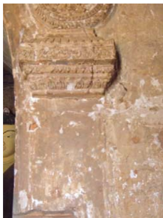
1457 MAHA-GU-GYI, VESTIBULE, WEST WALL, SOUTH SIDE. THE COLLAPSED PILASTER'S STUCCO PUT IN EVIDENCE THE FLAT FINISHING OF THE PLASTERING, THENCE NO PROPER ADHESION BETWEEN LAYERS.
