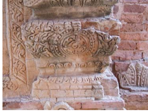
698 MONASTERY, HSIN-BYU-SHIN MONASTIC COMPLEX, FOREPART, WEST FACE, SOUTH SIDE. DRYING CRACKS OF STUCCO MOULDINGS. THESE ARE ALWAYS DIVIDED IN THREE LINES, CHARACTERISTIC TO LIME-BASED PLASTERS WHEN SETTING/DRYING.
