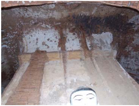
697 HSIN-BYU-SHIN-HPAYA, SOUTH CORRIDOR, INNER WALL. WATER INFILTRATION FROM ROOF DISSOLVING CONSTITUTIVE MUD MORTAR AND PLASTERS. NOTICE THE STRIPES OF BARE MASONRY.
