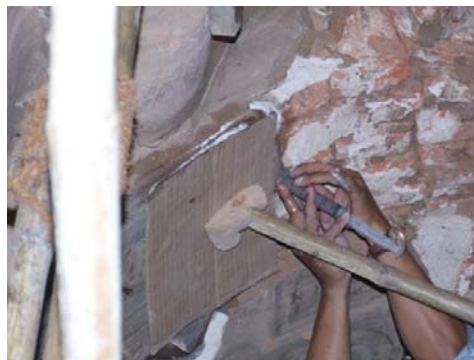
539 TAYOK-PYI-HPAYA-GYI, TEMPLE AT UPPER STOREY, SOUTH SIDE OF VAULT OF PASSAGE. GROUTING IS DONE THROUGH AN OPEN SIDE OF THE PLASTER.
