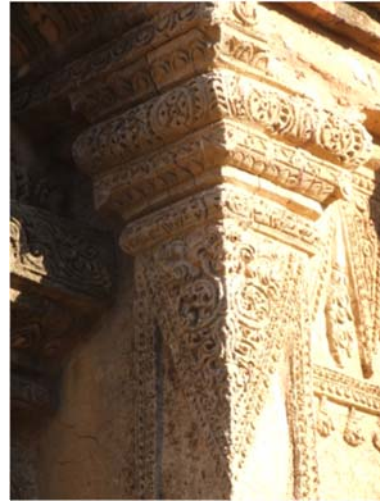
1152 TEMPLE. ERODED SURFACE DUE TO SLIGHTLY ACIDIC WATER RUN-OFF DISSOLVING CONSTITUTIVE MATERIALS.
