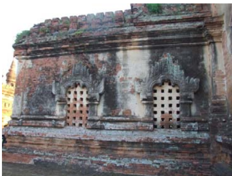
1085 SEIN-NYET-AMA, VESTIBULE EXTERNAL NORTH WALL. MICRO-ORGANISMS (FUNGI, ALGAE, LICHENS) DEVELOP ON DAMPENED
