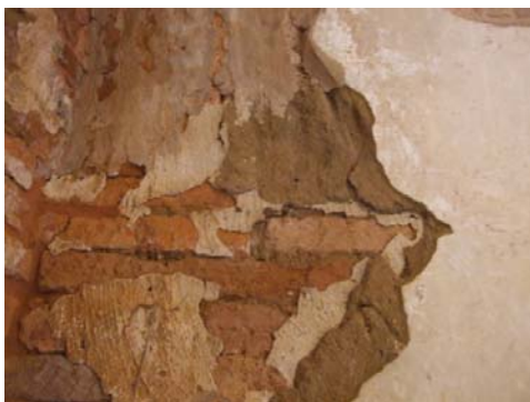
2119 TEMPLE. NOTICE THE ROUGH SPREADING OF THE LAYER OF LIME-BASED RENDERING, ON THIS, THE MUD PLASTER WAS APPLIED AND FINALLY COVERED BY THE THIN LIME-BASED PLASTER.
