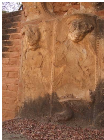
2162 ANANDA-OK-KYAUNG MONASTERY, PLATFORM RETAINING WALL, EAST FACE, SOUTH SIDE. INCISED CONTOURS FOR THE APPLICATION OF STUCCO.
