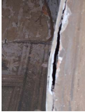
1460 TEMPLE, SHRINE, NORTH WALL, WEST SIDE. DETACHMENT WITH DEFORMATION OF PAINTED PLASTER.
