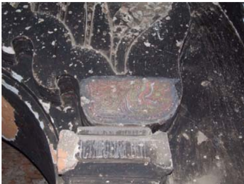
1668 SHWE-THI-HSAUNG, VESTIBULE, NORTH SIDE OF ARCH. CLEANING TEST WITH HEAVY DRIPPING BELOW. IT IS DIFFICULT TO GET RID OF THE LINES PRODUCED SINCE SOME ARE STILL DIRTY AND OTHERS OVER-CLEANED THUS, AN UNEVEN SURFACE IS CREATED.
