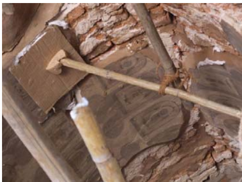
539 TAYOK-PYI-HPAYA-GYI, TEMPLE AT UPPER STOREY, VAULT OF PASSAGE TO SHRINE, SOUTH SIDE. MURAL PAINTINGS SEPARATED FROM THE VAULT ARE PROPPED BEFORE GROUTING.
