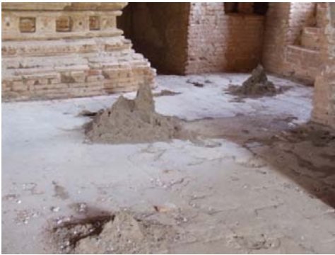
2128 TEMPLE. TERMITE NESTS IN THE ORIGINAL SANDSTONE SLABS FLOORING.
