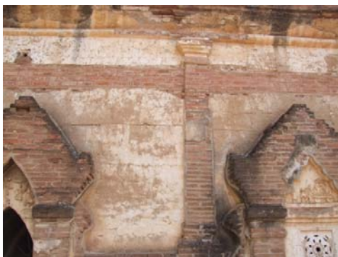
2162 ANANDA-OK-KYAUNG MONASTERY, WEST WALL, RENDERING WAS APPLIED FROM TOP TO BOTTOM IN SUCCESSIVE HORIZONTAL AND VERTICAL SECTIONS FOLLOWING PROBABLY, THE HEIGHTS OF SCAFFOLD.
