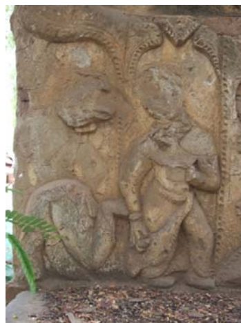
2162 Ananda-ok-kyaung Monastery. Yellow-brownish deposition on stuccoes as formation of a mixture of Calcium carbonate and dust.
