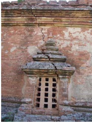
1249 PHYA-SA-SHWE-GU, CROSSING CRACK ALONG AND THROUGHOUT THE STRUCTURE.
