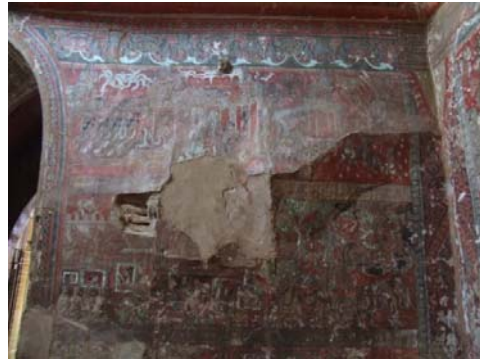
2007 SHWE-KYAUNG-U-HPAYA, WEST WALL, NORTH SIDE. DEFORMATION CAUSED TO THE ORIGINAL PLASTERS BY THE HARD FILLING IN CEMENT THAT DID NOT ALLOW ADJUSTMENT.
