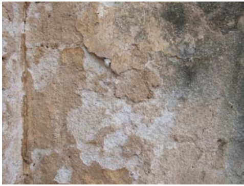
2162 ANANDA-OK-KYAUNG MONASTERY, PLATFORM RETAINING WALL, NORTH FACE, EAST SIDE. PLASTER LACKING COHESION (POWDERY) AND THIN LAYER OF WHITEWASH LACKING ADHESION.
