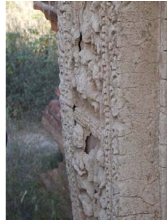
698 MONASTERY, HSIN-BYU-SHIN MONASTIC COMPLEX, FOREPART, WEST FACE, NORTH SIDE. STUCCO MOULDINGS SEPARATED FROM SUPPORT WITH STRONG DEFORMATION (BULGING).
