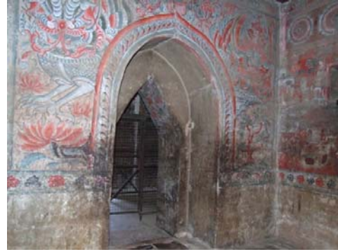
2162 ANANDA-OK-KYAUNG. GRIME AT HAND REACH AND FIXATIVES OBLITERATE THE PAINTED SURFACE AND CAUSED DETACHMENT OF PAINT (THE WHITE POINTS).
