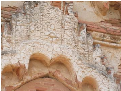
1498 NYA-PYA-GU, NORTH PORCH, PEDIMENT. WATER PERCOLATION ON SURFACE HAS
