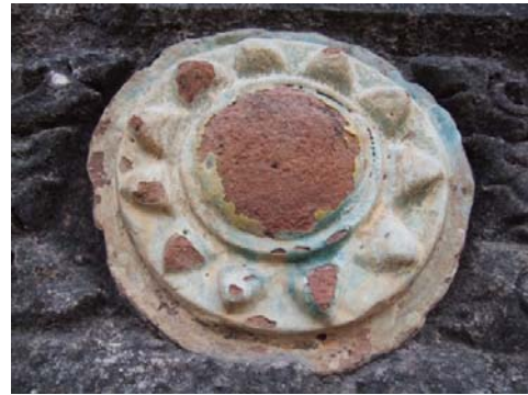
748 SULA-MANI-GU-HPAYA. GLAZED SANDSTONE ELEMENT. THE GLAZING, HAS DETACHED DUE TO ENVIRONMENTAL FACTORS AND LACK OF MAINTENANCE.
