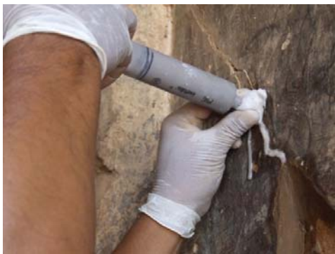
1580 LOKA-HTEIK-PAN, PORCH, EAST WALL. DURING A GROUTING TEST WITH MATERIALS LOCALLY FOUND SUCH AS SLAKED LIME PUTTY, POZZOLAN, JAGGARY.
