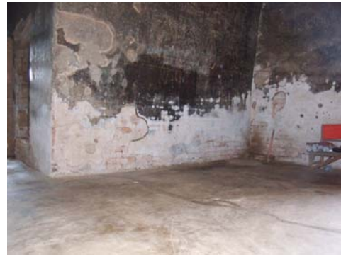
1605 PATHO-HTA-MYA, VESTIBULE, SOUTHEAST CORNER. RISING WATER DUE TO A POND-LIKE AROUND THE TEMPLE DURING THE RAINY SEASON. THE PROBLEM WOULD OBVIATE IF REMOVING SOME SOIL FROM THE ROAD AT THE NORTH WEST FOR WATER EVACUATION.
