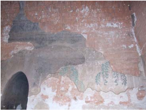
537 TAYOK-PYI-HPAYA-GYI, VESTIBULE, NORTH WALL. THE DARK BROWNISH AREA ABOVE THE ARCH IS A FORMER FILLING WITH MUD-BASED PLASTER AND THEN PAINTED FOR COMPLETING THE LOST DECORATION.
