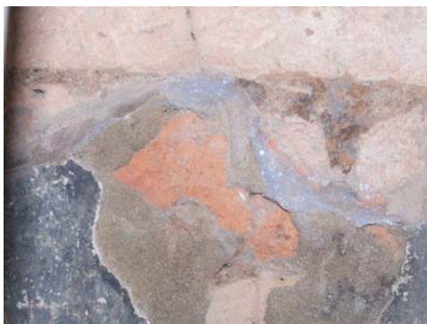
1600 NAT-HLAUNG-KYAUNG. MUD-BASED PLASTER & LIME-BASED PLASTER.
