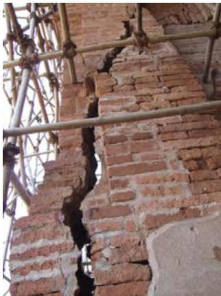
539 TAYOK-PYI-HPAYA-GYI, 1 ST FLOOR, WEST PORCH, CROSSING CRACKS THROUGHOUT THE MASONRY.
