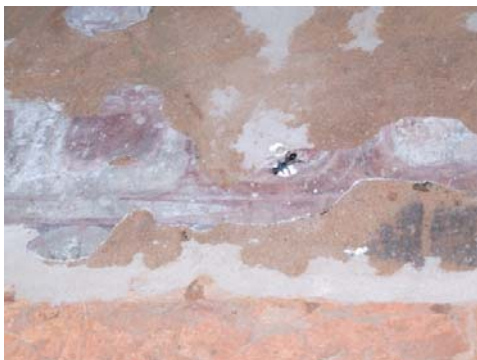
1323 KUBYAUK-GYI (MYINKABA), VESTIBULE, SOUTH WALL. INSECT EATER OF ACRYLIC RESINS
