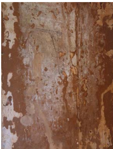
474 TEMPLE. MUD-BASED PLASTER & WHITE PRIMING LAYER.
