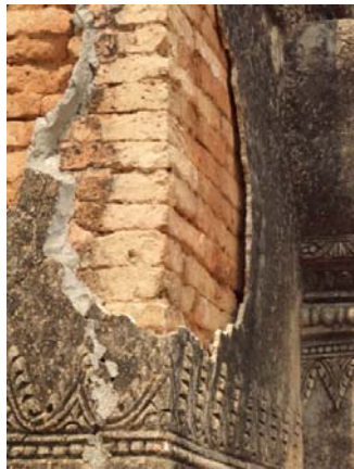
1467 LOKA-OK-SHAUNG, UPPER STOREY, PORCH, SOUTHEAST CORNER. DEFORMED RENDERING DUE TO THERMAL EXPANSION & CONTRACTION.
