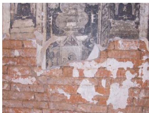
1847 TEMPLE, HPAYA-NGA-ZU GROUP. LIME-BASED PLASTER – 3 LAYERS.
