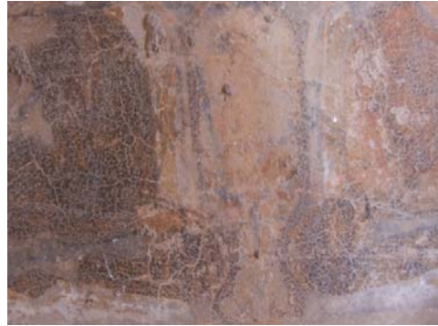
539 TAYOK-PYI-HPAYA-GYI, UPPER STOREY TEMPLE, VESTIBULE, NORTH WALL. DETAIL OF PAINTING, PROBABLY A PURPLE LAKE, WITH EVIDENT CRAZING DUE TO EXCESSIVE WEATHERING.
