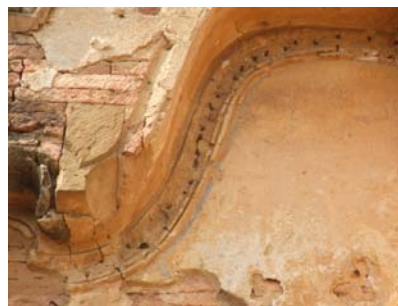
1812 HTI-LO-MIN-LO TEMPLE, EAST FACE, SOUTH SIDE. WOODEN PEGS INSERTED INTO THE MASONRY AND RENDERING THAT SUPPORTED DISAPPEARED STUCCO MOULDINGS. NOTICE THE PAINTED BANDS THAT MIGHT HAVE FORMED PART OF A LOST DECORATIVE CYCLE.
