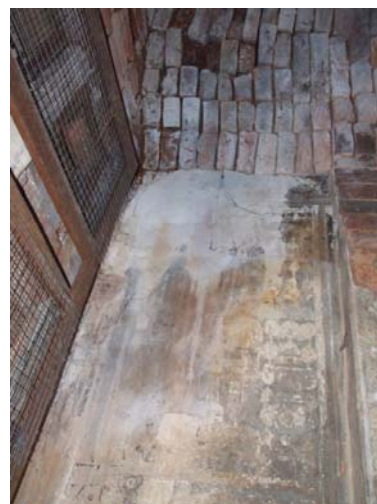
1323 KUBYAUK-GYI (MYINKABA), NORTH LATERAL FOREPART WITH WINDOW, EAST SIDE, INDOORS. WATER INFILTRATING HAS OBLITERATED THE UPPER SECTION OF MURAL PAINTING. THE WHITE AREAS CORRESPOND TO DRY MASONRY WITH RE-CRYSTALLISED SALT.
