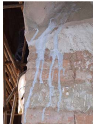
539 TAYOK-PYI-HPAYA-GYI, FIRST STOREY TEMPLE, SOUTHEAST CORNER OF CENTRAL CORE IN SHRINE. GROUTING MATERIAL RUN-OFF OVER THE SURFACE THAT WAS NOT REMOVED SO THIS WILL SHOW FOREVER A WHITE INDELIBLE STAIN. IT IS IMPORTANT TO BE ATTENTIVE.
