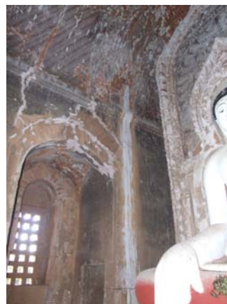
997 KYAUNG-GYI-NIMA (AMA). SHRINE, SOUTH WALL. THE WHITE LEAKAGE OF GROUT CORRESPOND TO A FORMER LEAKAGE OF MUD MORTAR. THE MASONRY REPAIR TEAM WAS UNAWARE OF THE PROBLEM SO NOT UNDERTOOK THE NECESSARY MEASURES TO PUT REMEDY.
