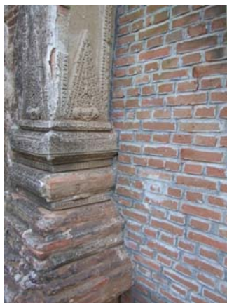
997 KYAUNG-GYI-NIMA (AMA), WEST PORCH, NORTH. THE BUTTRESS FOR SUPPORTING THE PORCH WAS BUILT WITH STRONG CEMENT DIRECTLY ON THE STUCCO MOULDINGS WITHOUT ANY PROTECTION OR BUFFER. ATTENTION TO STRUCTURAL WORKS BE AWARE!!!
