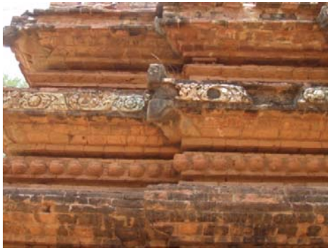
1145 SO-MIN-GYI-HPAYA, EAST SIDE. CALCIUM CARBONATE DEPOSITIONS ON GLAZED PLAQUES AS WELL AS BLACK DEPOSITS FROM ALGAE ON THE ROUGH SECTIONS WITHOUT GLAZING THAT DEVELOP DURING THE RAINY SEASON.
