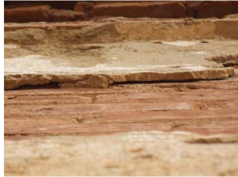
2162 ANANDA-OK-KYAUNG MONASTERY, NORTH FACE, SEPARATED RENDERING FROM THE WALL
